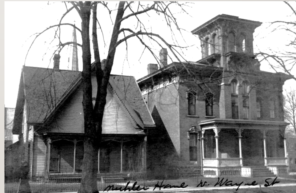
CHARLES F. MUHLER HOUSE (RIGHT) PHOTO, C.1935
