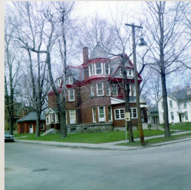
R.W.T. DEWALD HOUSE (ROCKHILL HOUSE IN BACKGROUND) C.1962
